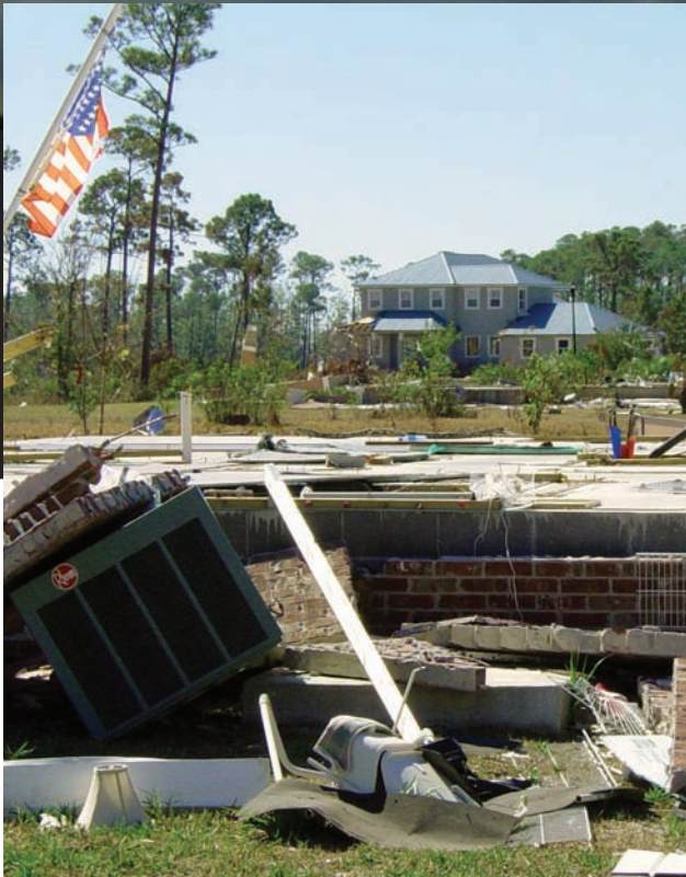
Every home in this neighborhood was destroyed by a category 5 hurricane, except the one built with ARXX ICFs.
